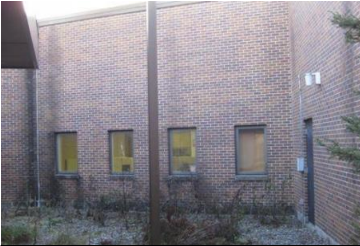
Photo #4: Overview of north elevation and windows.
