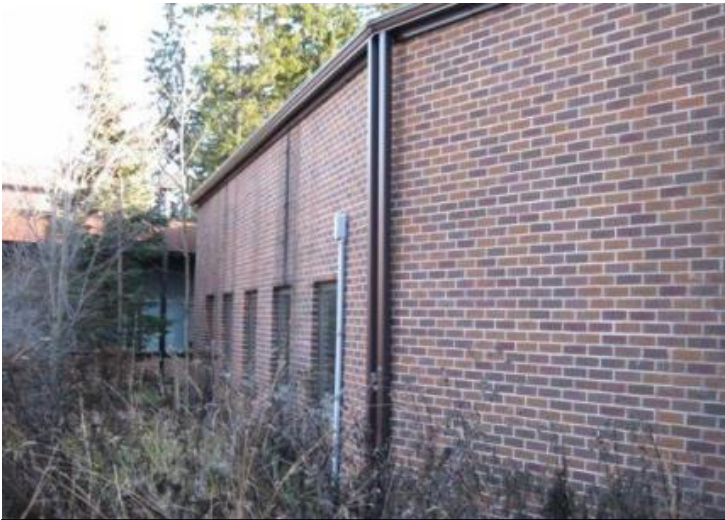
Photo #5: Overview of north elevation.
