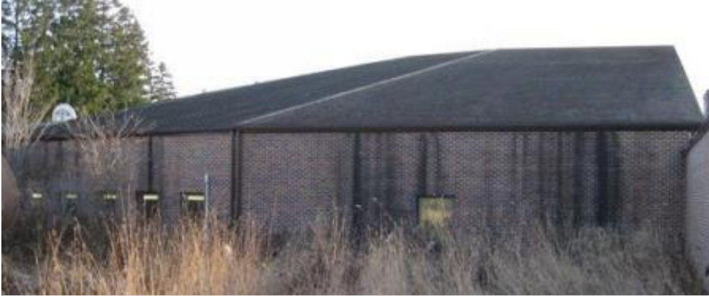
Photo #1: Overview of Roof Area I3 and subject wall.
