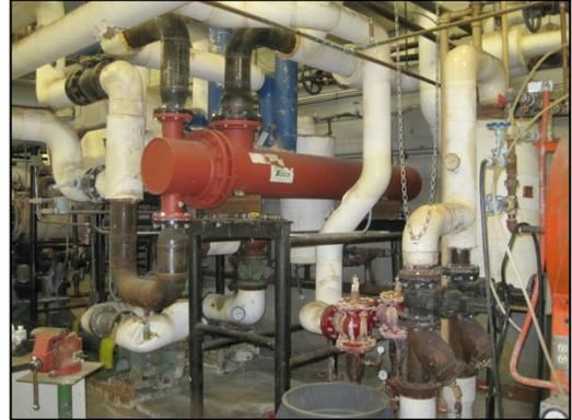
Existing Steam Heat Exchangers and Steam and Condensate Piping will be replaced
