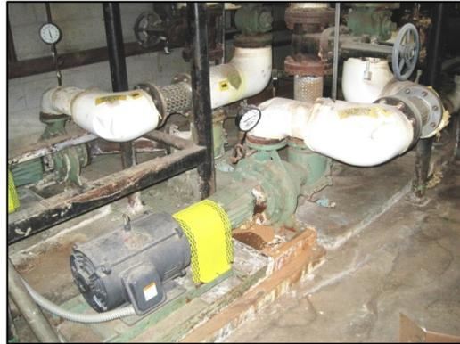
Pump and Boiler Concrete pads will need to be removed
