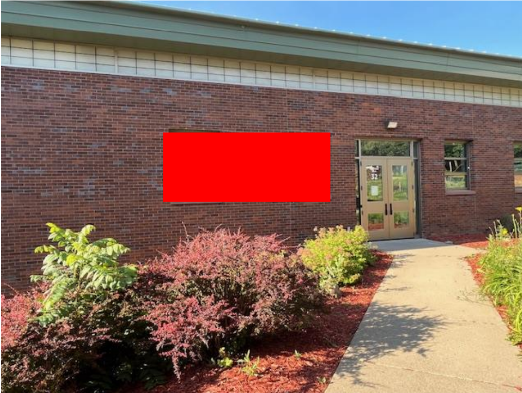
Figure 3 – Existing wall elevator with proposed location of new artwork highlighted
